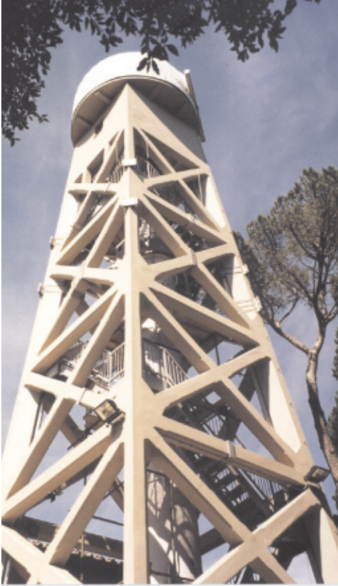
Top: The Solar Tower, Firenze
